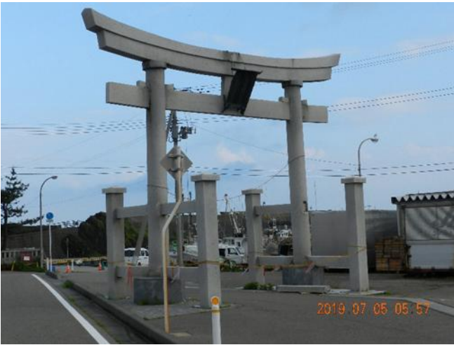
Fig. 7 Damage due to the earthquake rocked at June 18, 2019. Destruction of the torii (stonework) of "Itsukushima Jinjya (Shintou shrine)" in Nezugaseki, Tsuruoka City, Yamagata Prefecture (photo in July 5, 2019). The location of the torii is given in Fig. 5.
