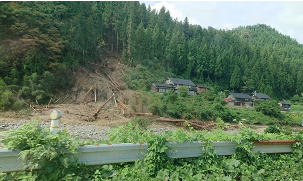
Fig. 6 An area damaged by heavy rain in Nishiwaki-machi, Wajima City, along Prefectural Route 1 (Fig.1-a-⑤).
