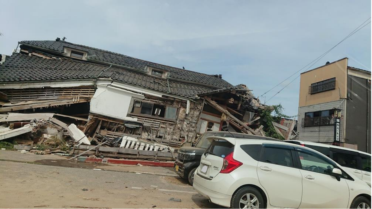
Fig. 10 Houses collapsed in Wajima City due to earthquake. Located in Kawai-machi, Wajima City (Fig.1-A-⑨).
