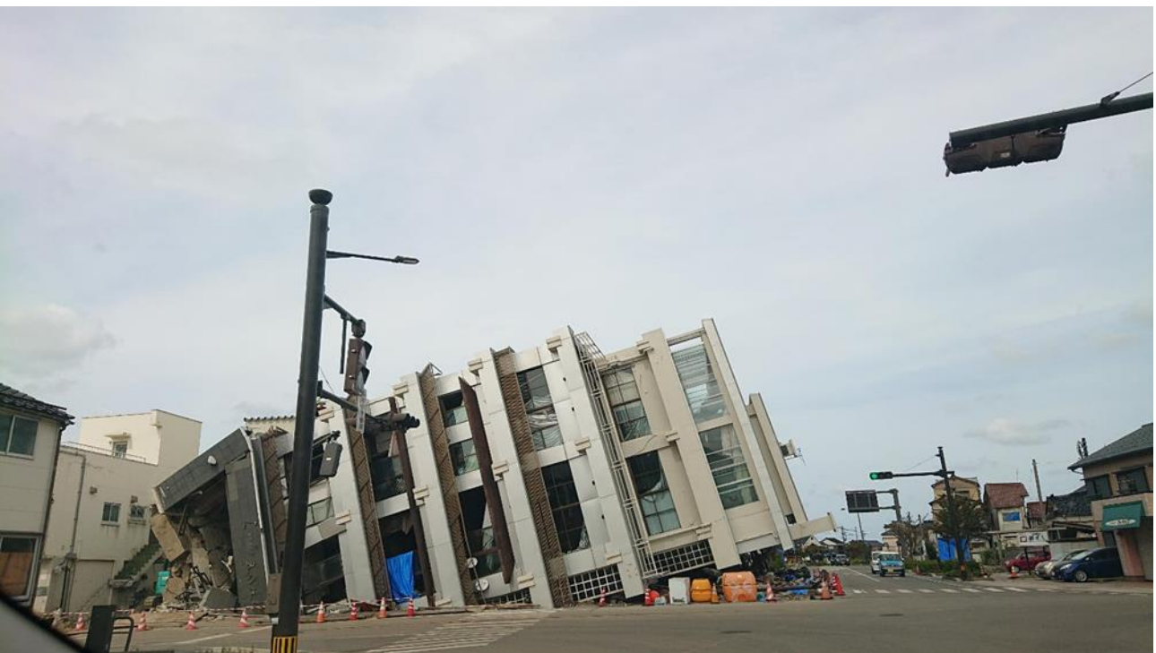
Fig. 11 Scenes of a collapsed building in the center of Wajima city. The traffic light tilted due to the earthquake. The photo shows the Goshimaya Building in Kawai-machi, Wajima City (Fig.1-a-⑩).
