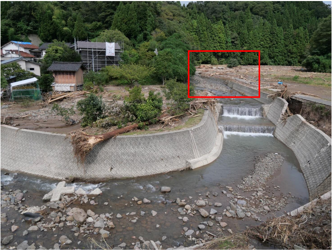
Fig. 7a Driftwood from the mountains and traces of a flooded river caused by heavy rain in Zouda, Ishiyasumiba-machi, Wajima City (Fig.1-a-⑥).
