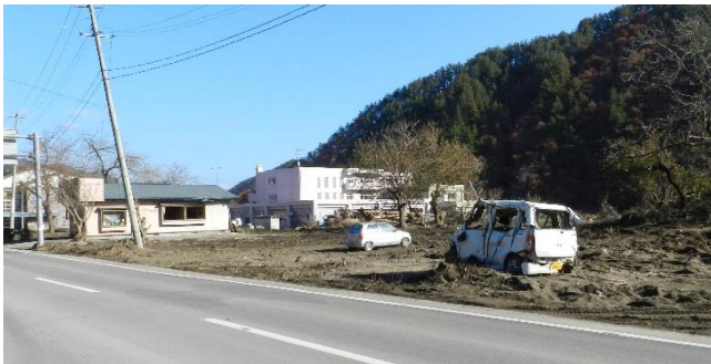
Fig. 11 Inundated area along National Road 455 at Otomo in Iwaizumi Town (photo in Nov.14, 2016). A seriously damaged car by the flooding and a flooded wooden house. The building in back is the nursing facility of Fig. 9.
