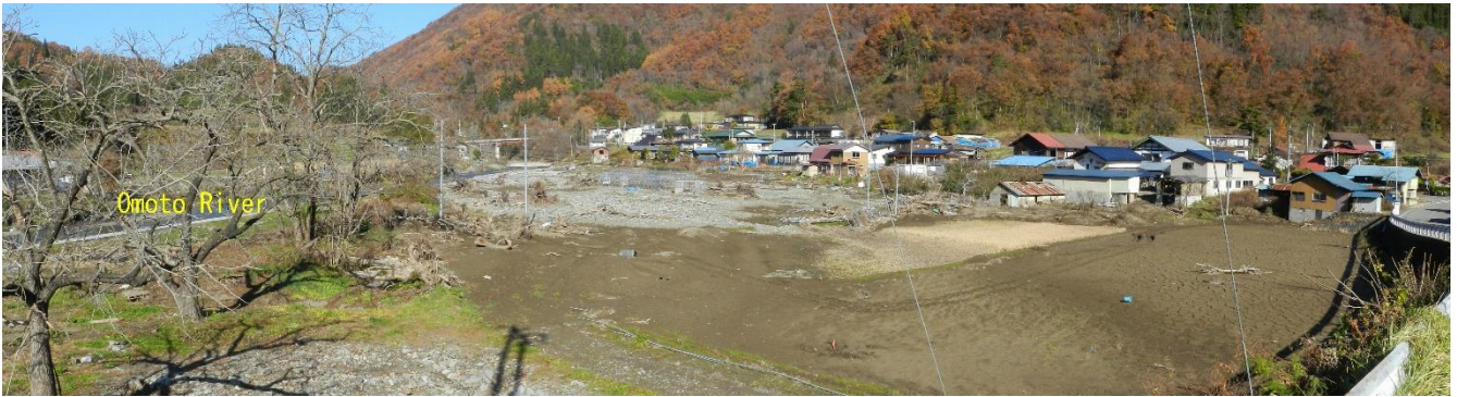
Fig. 5 Damage of agricultural land by the flooding at slightly upper reach of the Anazawa Bridge of the Omoto River, in Iwaizumi Town (Loc. D of Fig. 1). The road which consists of fill is approach of the bridge. Photo in Nov.14, 2016.
