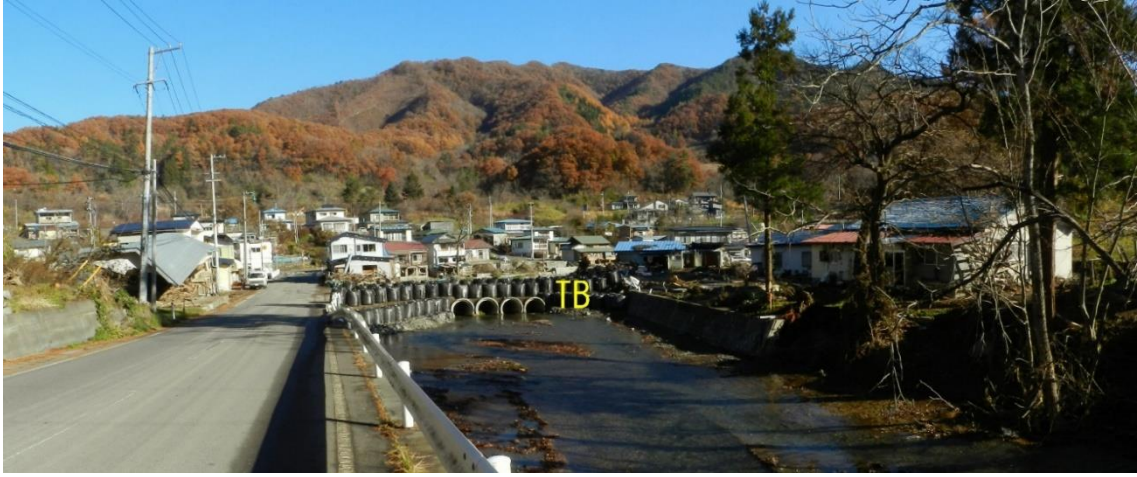
Fig. 4 Destruction of wooden houses by the flooding along the Mitakai River at Nameiri, in Iwaizumi Town (Loc. B of Fig. 1). TB: Temporary bridge. Photo in Nov.14, 2016.
