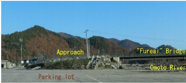
Fig. 10 "Fureai" Bridge and its approach which consists of filling at Otomo in Iwaizumi Town (photo taken from the upper stream in Nov.14, 2016). The face of slope was eroded and the guardrail was broken by the flooding.
