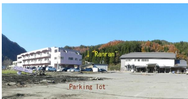
Fig. 9 Inundated area of Otomo in Iwaizumi Town (photo in Nov.14, 2016). Flooded buildings, two nursing facilities for elderly people and dairy company (from the left to the right).
