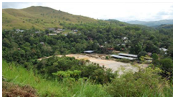
Fig. 4 A view of Ga'ang community (photo courtesy of the Mines and Geosciences Bureau)
